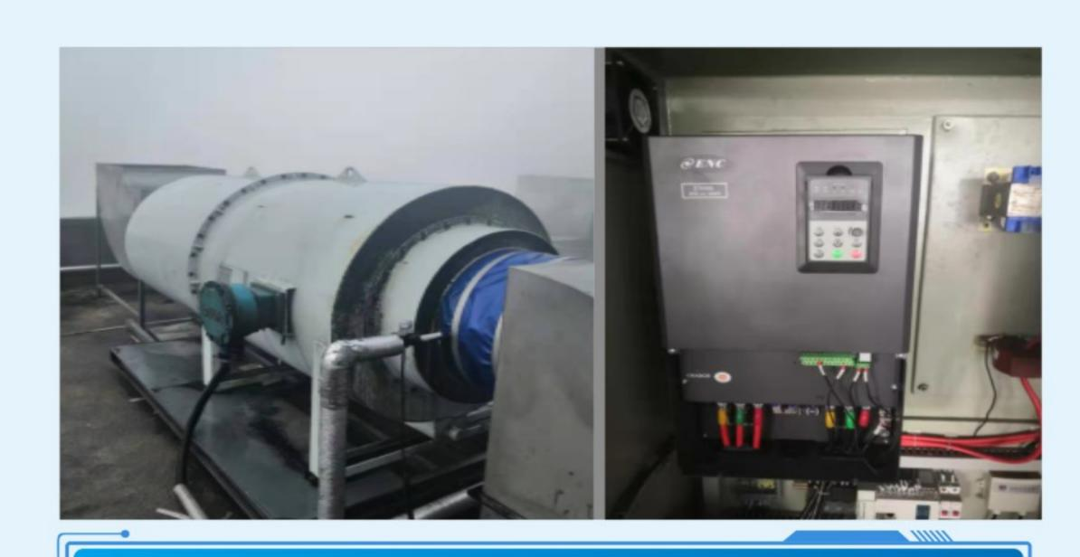
Coal washing plant drying system, using 6 units of EN600-7T series inverters on site
