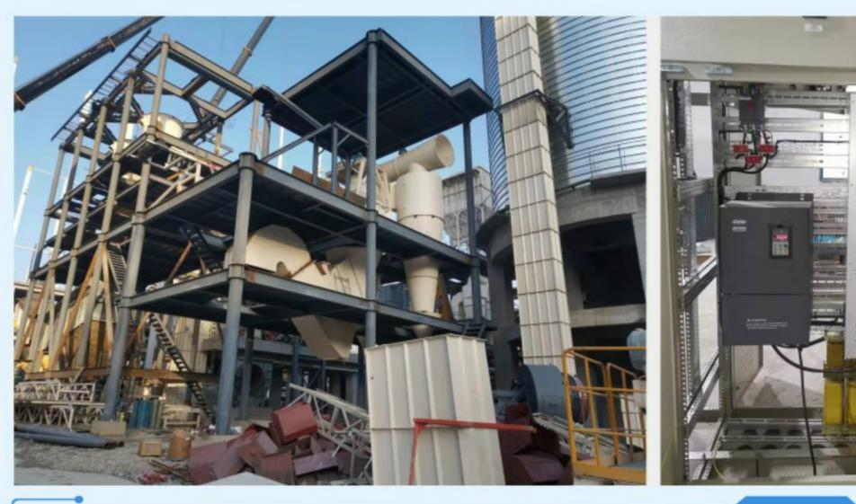
Powder dressing machine, using EN500 inverter + EN550 active front end
