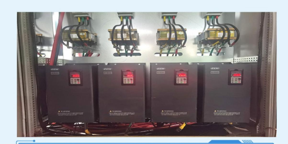
Seamless steel pipe sizing machine, 14 units of EN600 series inverters are used on site
